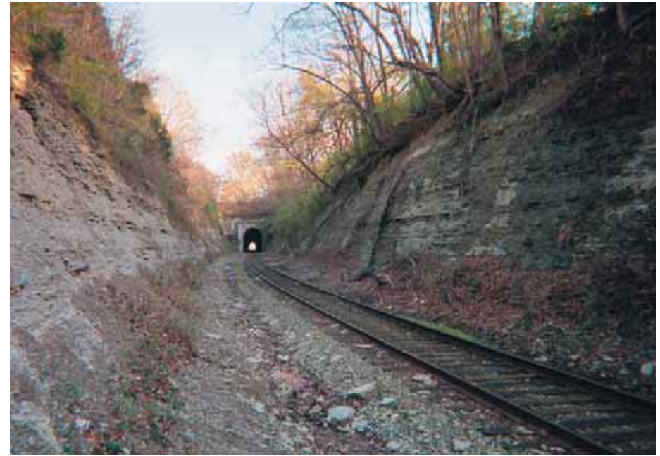
Rail Road Tunnel
